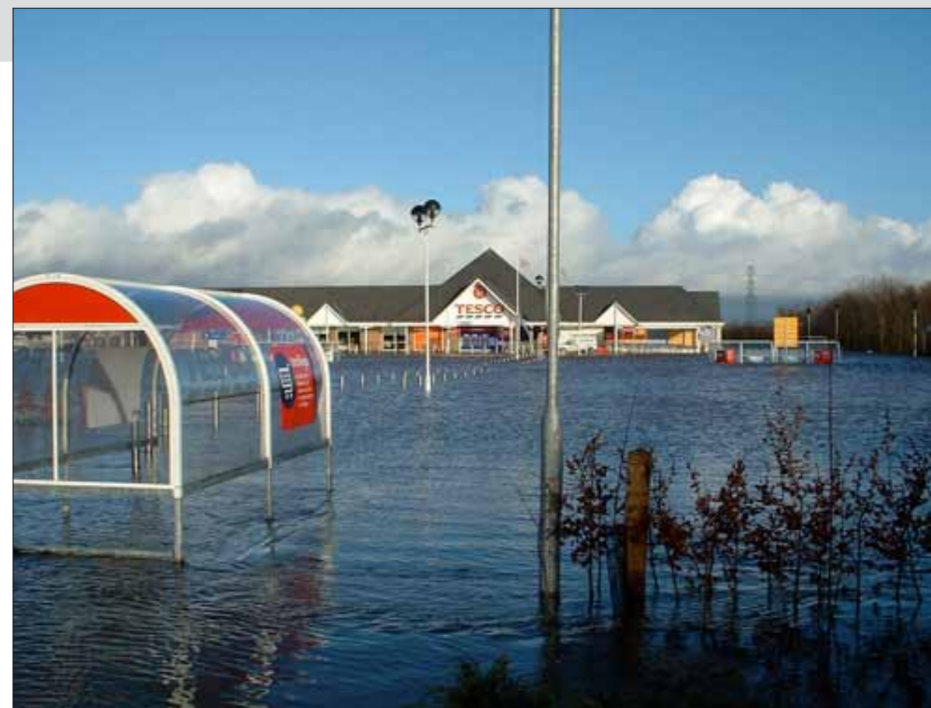
A Tesco store flooded after heavy rains.
